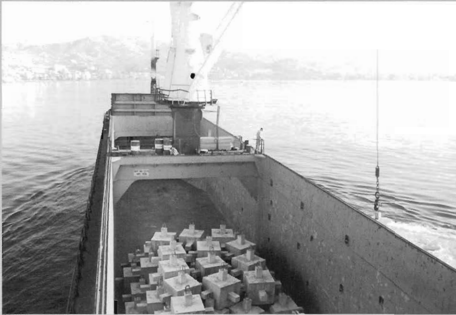
Installation of artificial reefs
