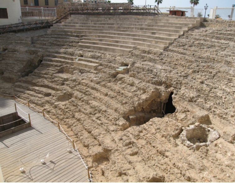
General view of the seating area
