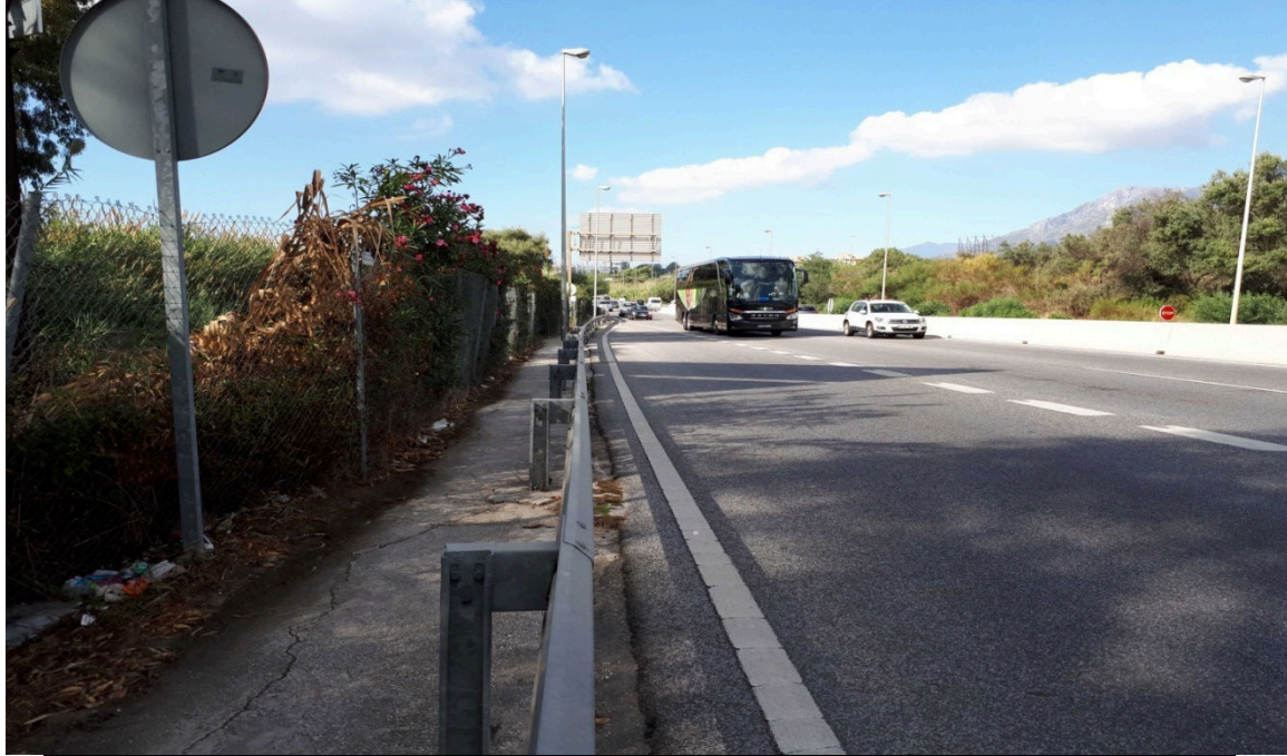
Picture no 1 Section no 6 Km 7-11 4 km of heavy traffic on the route (national road number N340/A-7). Without alternative.
