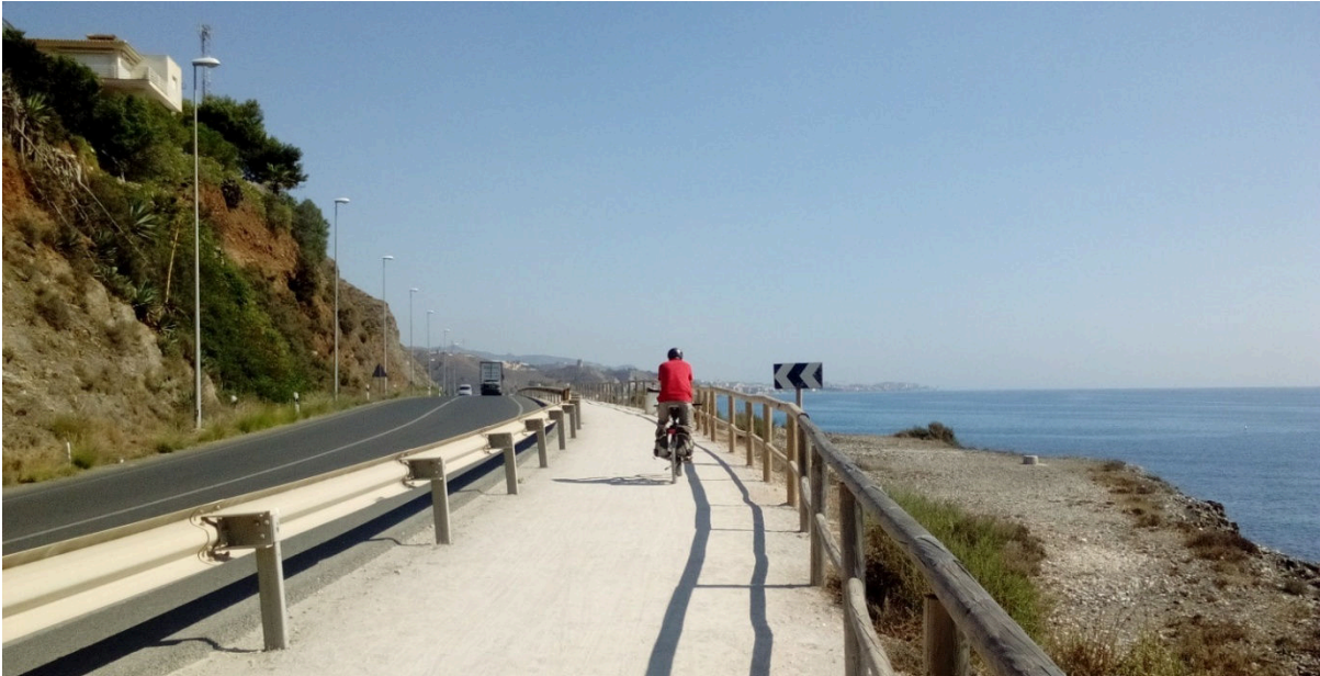
Path built on compacted soil, parallel to public road (Section 9)
