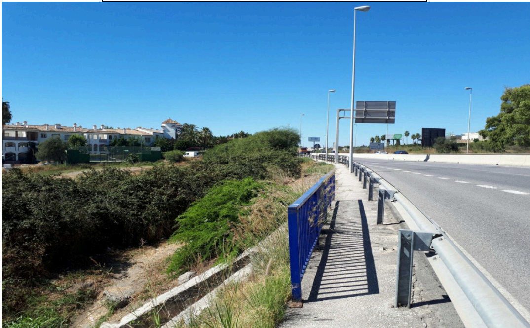
Picture no 1 Section no 5 Km 9 1.200 m of heavy traffic on the route (national road number A-7). Without alternative currently.
